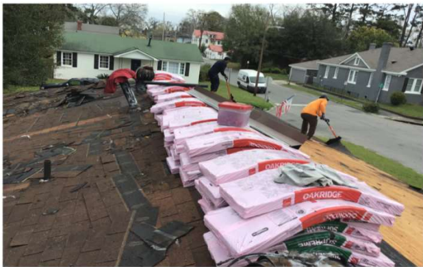
Homeowner Roof Replacements
